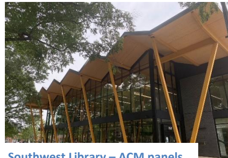
Southwest Library – ACM panels, Curtainwall and energy efficient glass.
