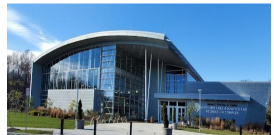
SARRC – Curtainwall, automatic entrances, custom interior glazing, exterior energy efficient glass and glazed in metal panels.
