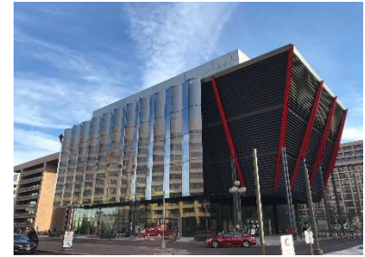
International Spy Museum – Custom steel and glass veil, Skylight, Returnwalls and soffit glass systems fabricated and furnished by Roschmann
